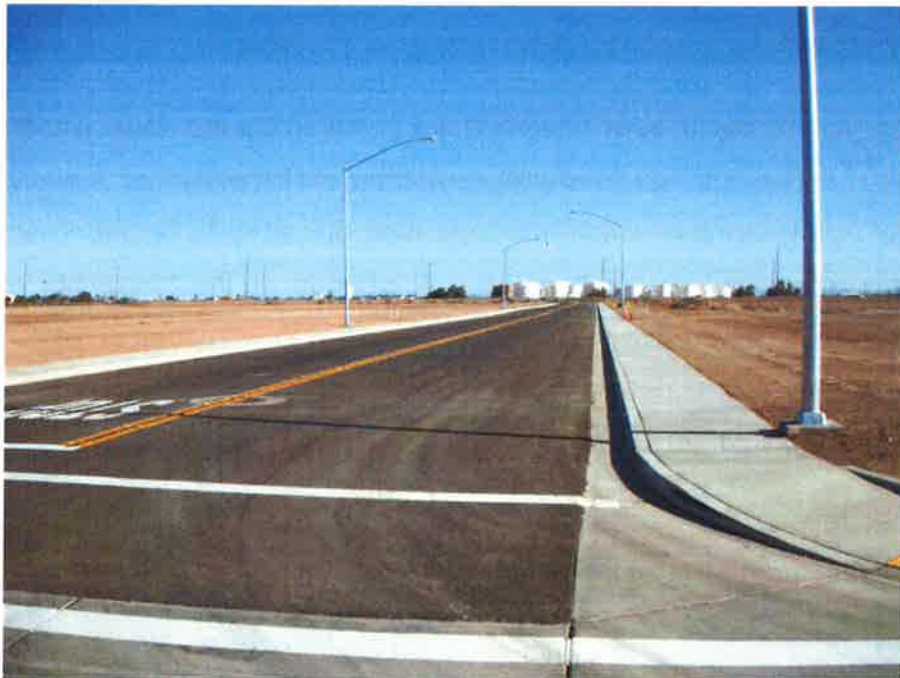
Figure 2 – 12 Street from the south (after picture)
