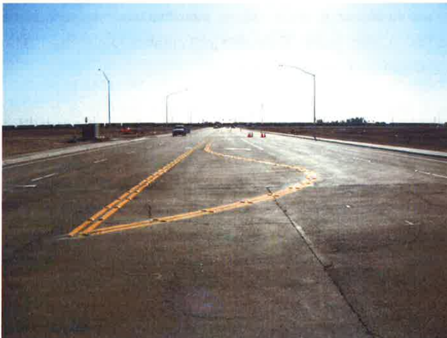
Figure 4 – Cruickshank Drive from the west – after picture
