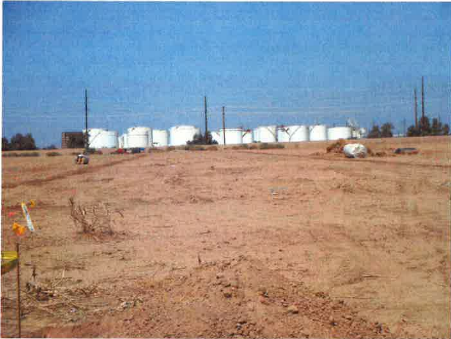
Figure 1 – 12 Street from the south (before picture)
