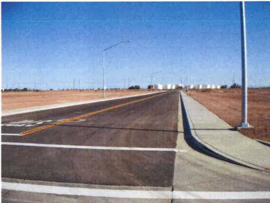
Figure 2 – 12 Street from the south (after picture)
