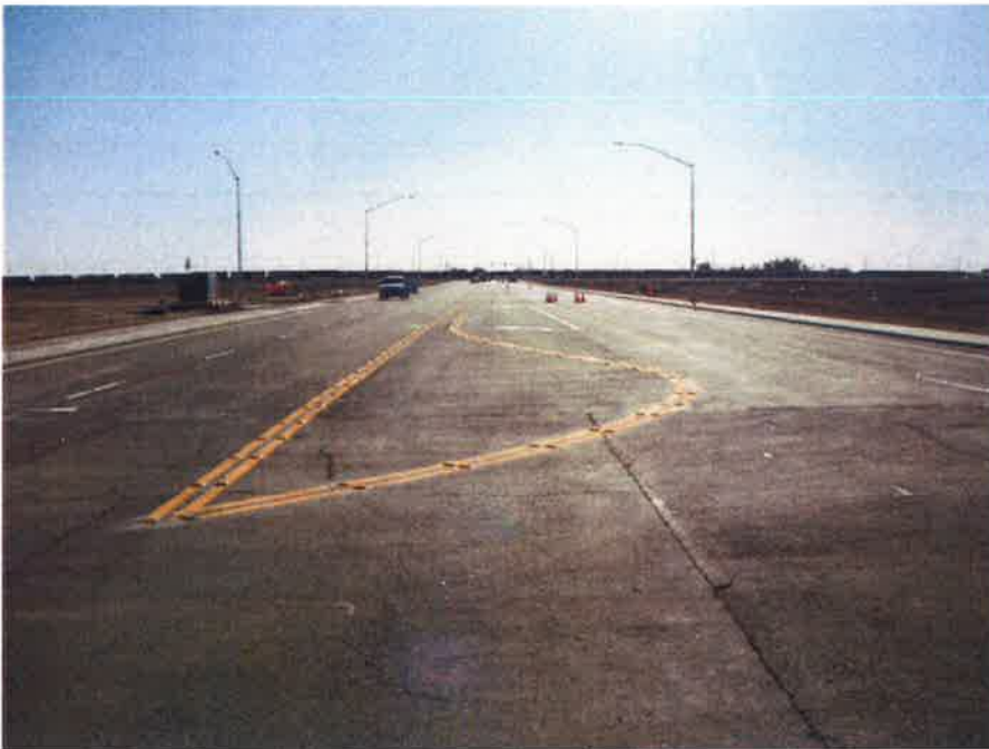
Figure 4 – Cruickshank Drive from the west – after picture
