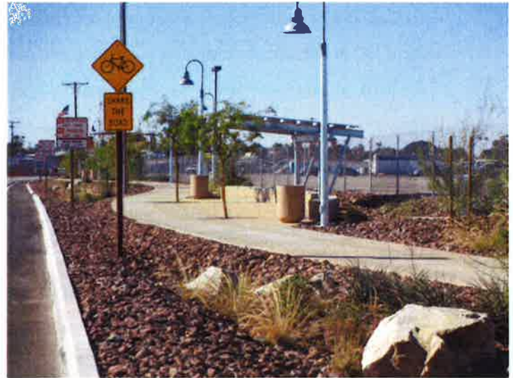
Caltrans Pedestrian Improvement Project at Andrade/Los Algodones POE
