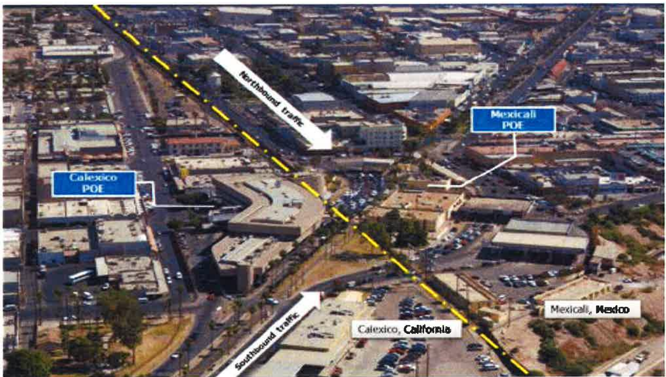
Existing Calexico West/Mexicali I POE
