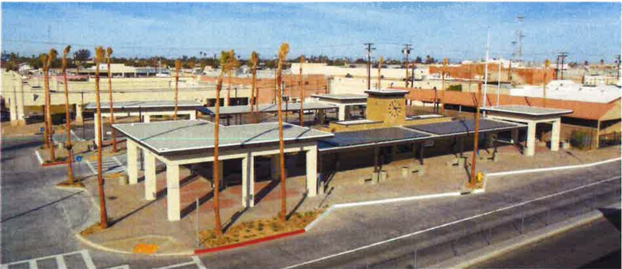
City of El Centro Transit Transfer Station
