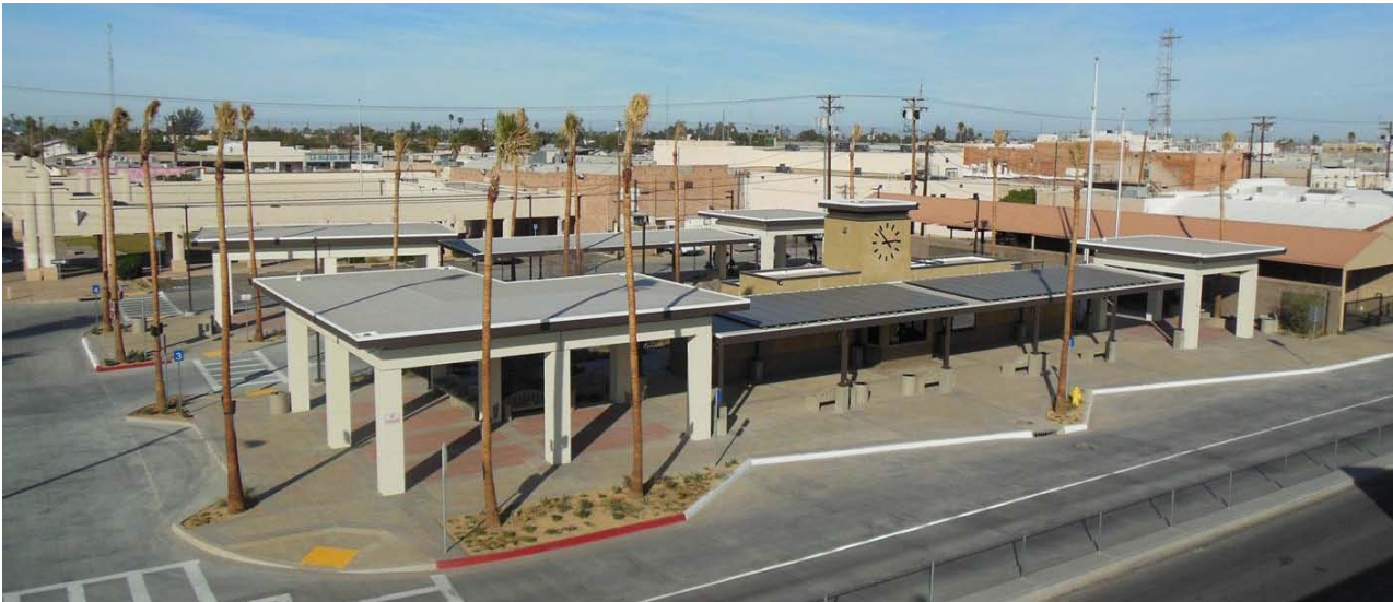
City of El Centro Transit Transfer Station
