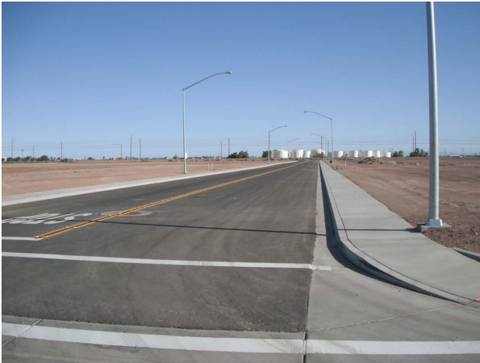
Figure 2 - 12 Street from the south (after picture)
