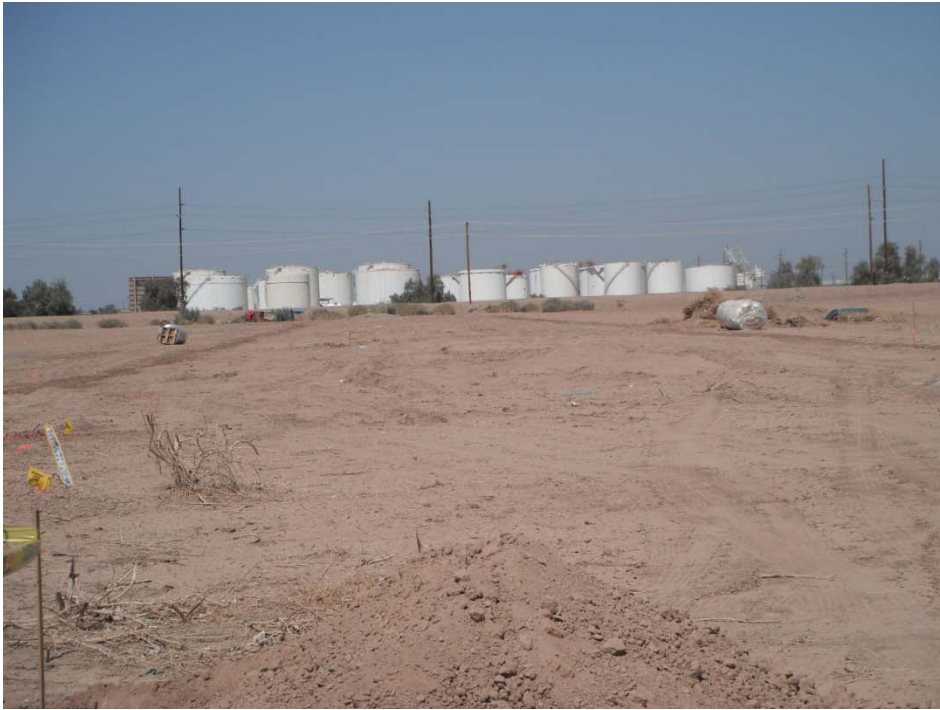
Figure 1 - 12 Street from the south (before picture)
