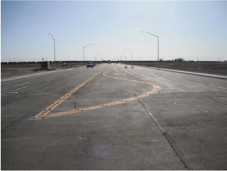
Figure 4 – Cruickshank Drive from the west – after picture
