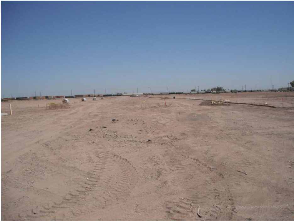
Figure 3 – Cruickshank Drive from the west – before picture
