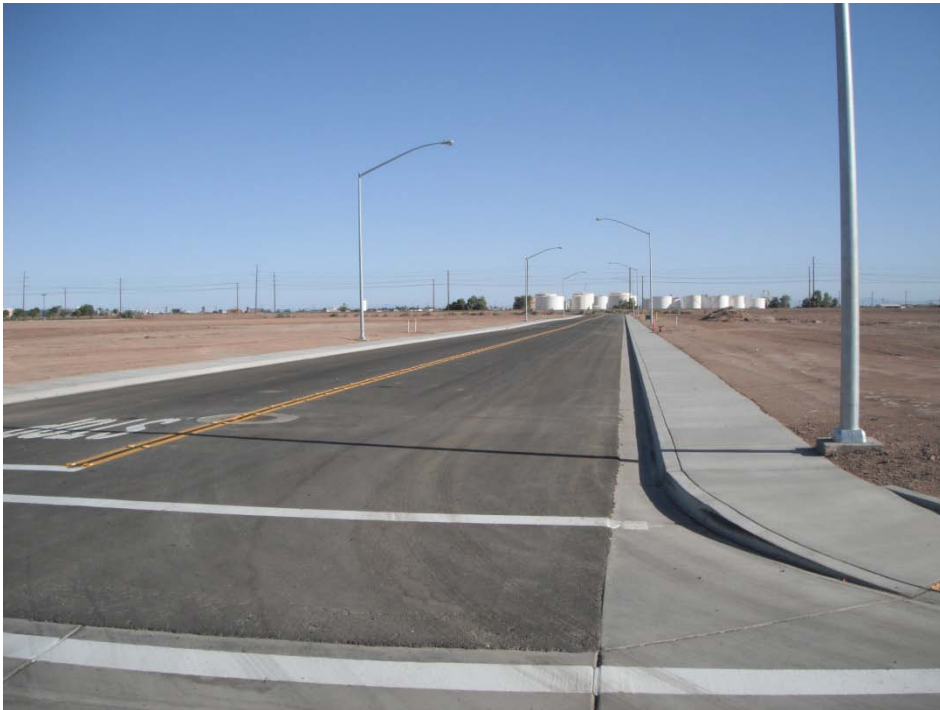
Figure 2 - 12 Street from the south (after picture)
